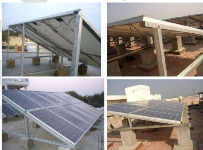
Figure 4.7: GI mounting structure
